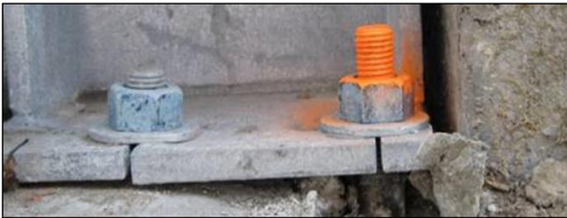
Full bolt depth required
