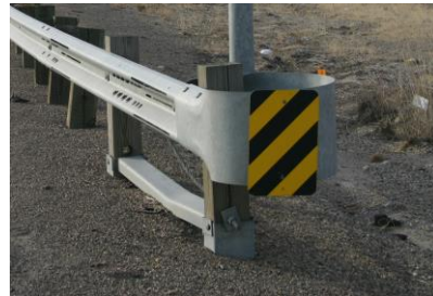
Missing Bearing Plate
