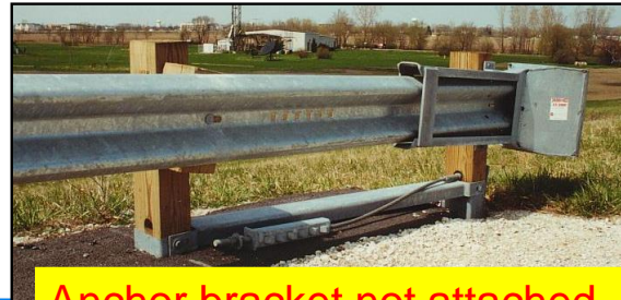
Anchor bracket not attached
