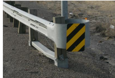
Missing Bearing Plate
