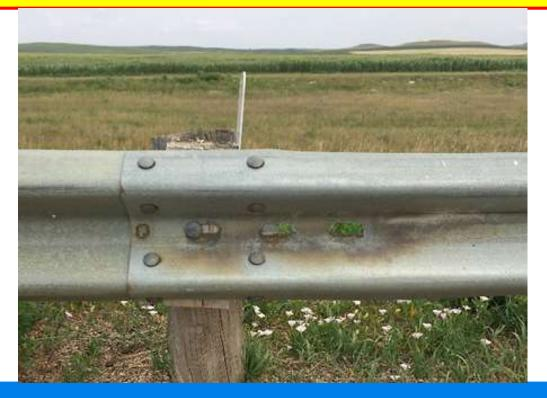
Using a torch on the rail element may compromise the strength of the rail.
