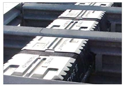
**Typical QuadGuard Cartridges**
