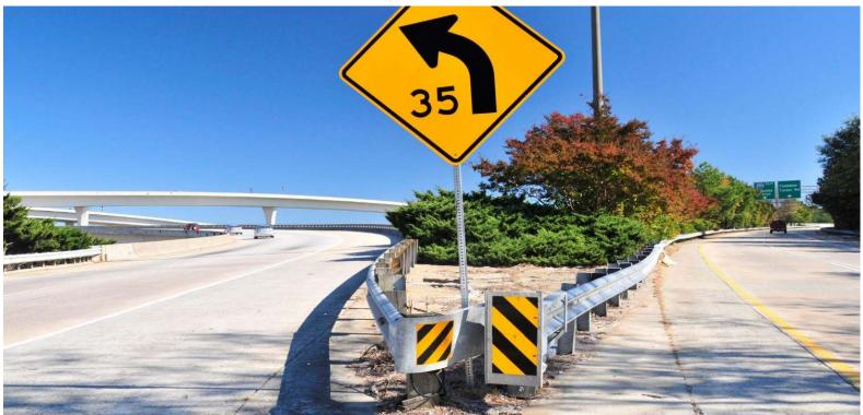
**Improper Application** – Terminals should have 7' separation (and the sign should be beyond the terminal system)
