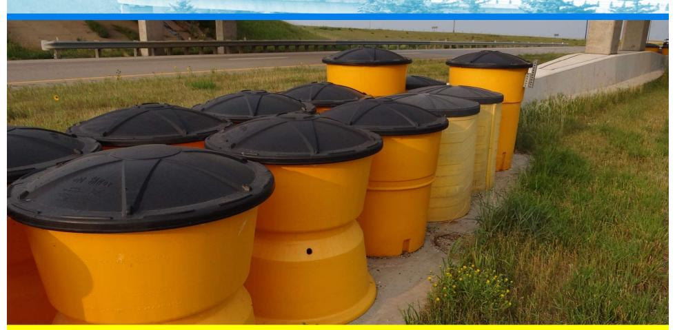
Place sand container in the correct position with the correct amount of sand.
