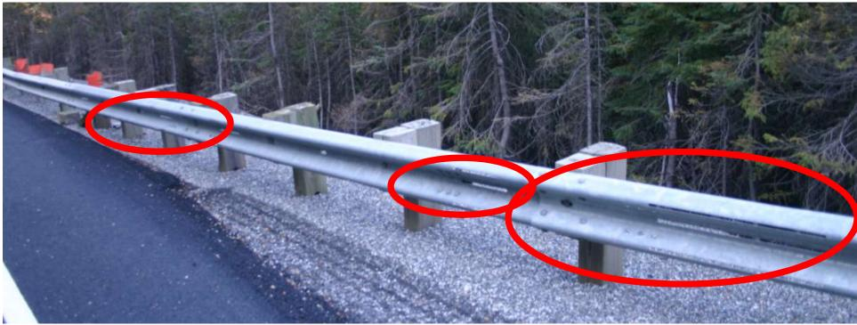
Whether construction or maintenance, never would have THREE slotted rails.
