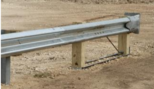
TxDOT Design 9'- 4 1/2 " rail element Rail ends at last post
