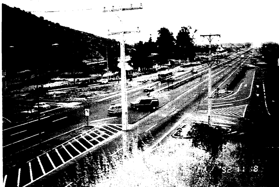
Figure 11: Some heavy volume facilities are beset with problems of left turn opportunities, and hazardous placement of roadside objects.
