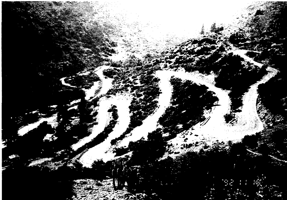
Figure 8: In mountain terrain, severe horizontal curves require adequate signing, delineation, and guardrail placement to help avoid run-off-road accidents.
