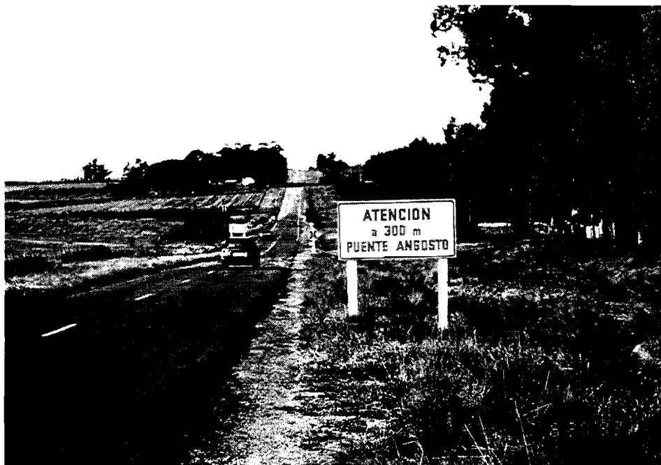
Figure 21: Roadside clear zone may be compromised by sign placement.
