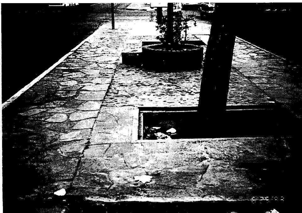
Figure 18: Even in instances where a pedestrian refuge is provided, hazards may be "built in". In this case the tree grows in a hole and can cause pedestrian injury.
