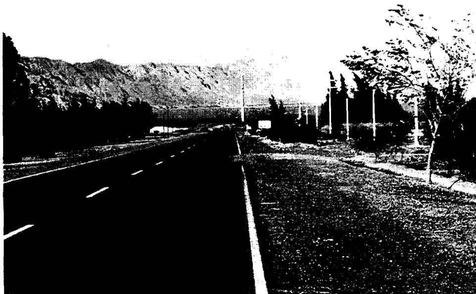
Figure 15: When an adequate clear zone is available on the roadside, there is a good chance that a motor vehicle can recover if it leaves the road.
