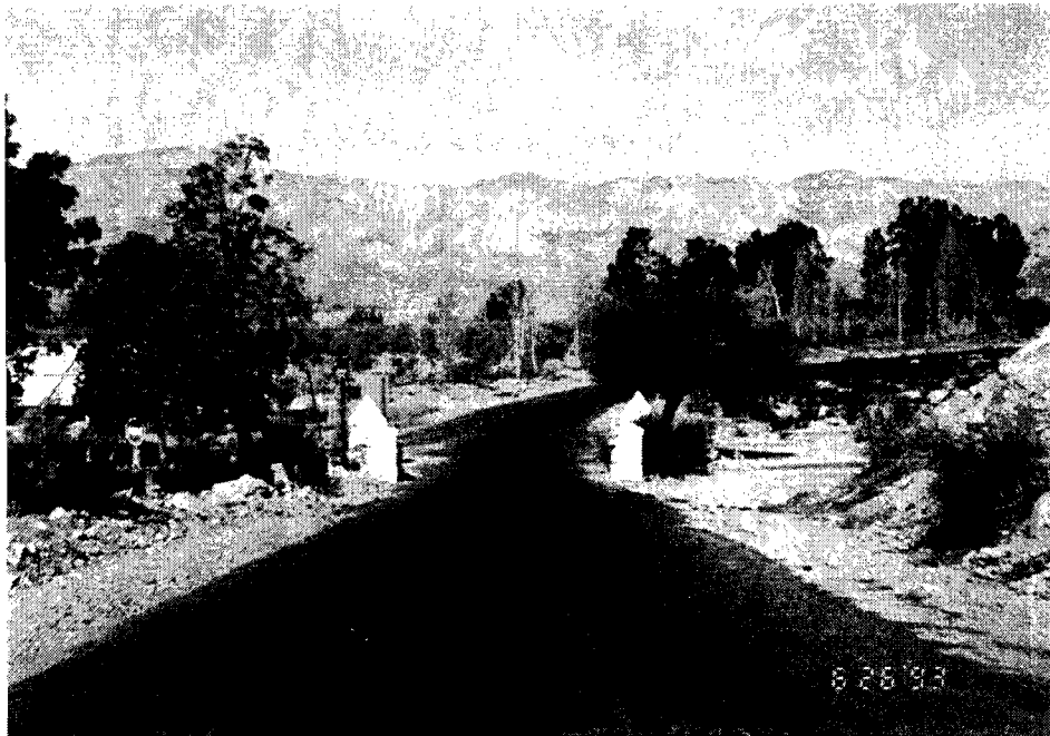
Figure 10: Narrow bridges abound in some rural areas and the hazard may be reduced only slightly by warning signs.
