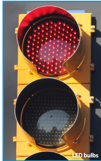
The HSRC study showed no significant decrease in safety, and one possible increase, when replacing incandescent bulbs in traffic lights with LED ones.
